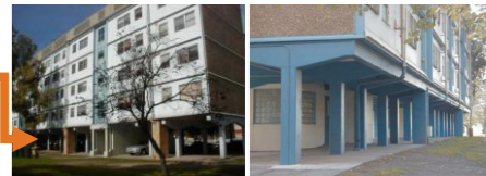
Figure 2: Soft storey building
